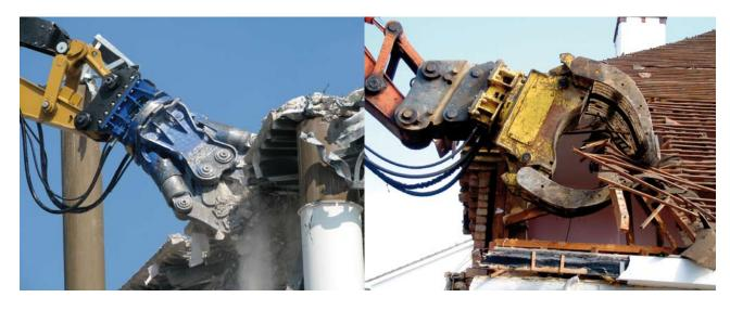
**Crusher for Primary Demolition:** Primary demolition of structures especially made from concrete or tile **Grapple Crusher:** Primary and secondary demolition of structures made from tile
